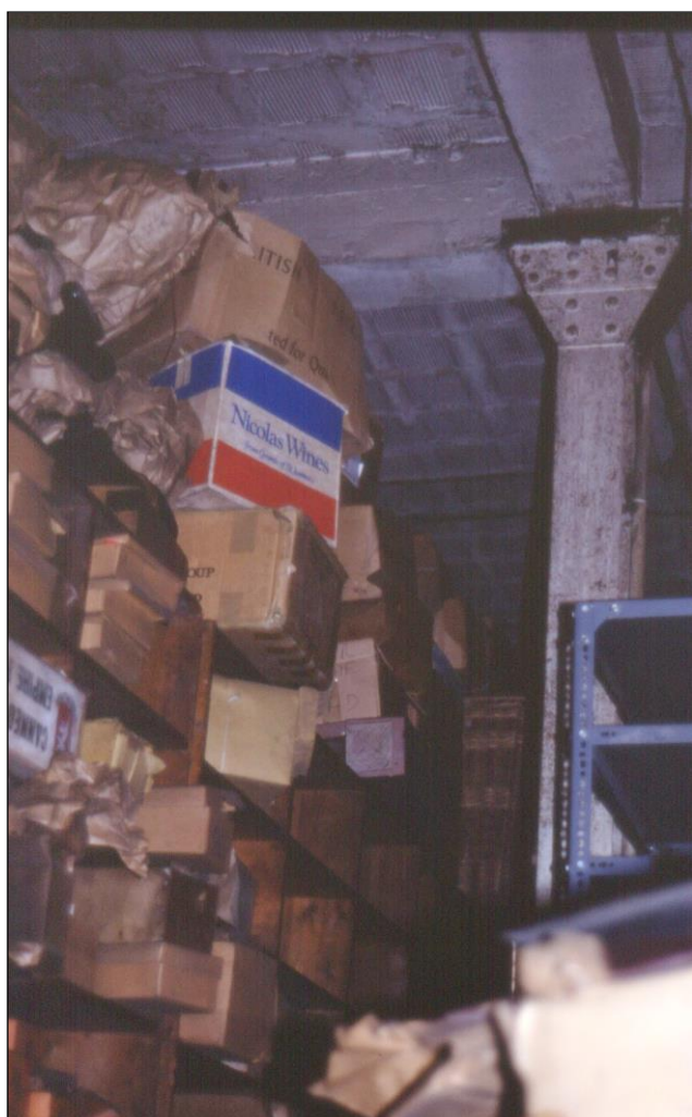
A view of the Crypt showing boxes stored up to the high ceiling.
