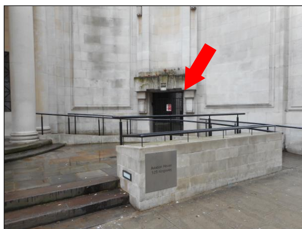
If you stand in front of the old church façade of Aviation House today (2016), you can still see on the right of the building the gateway (arrowed) which led down a staircase towards the Crypt.
